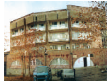
The Armenian American Wellness Center currently occupies the first floor of this building in Yerevan.
